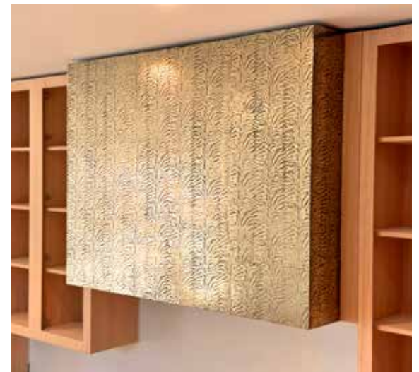
A metal skin application was used on the kitchen hood. Courtesy of Badilla Painters
